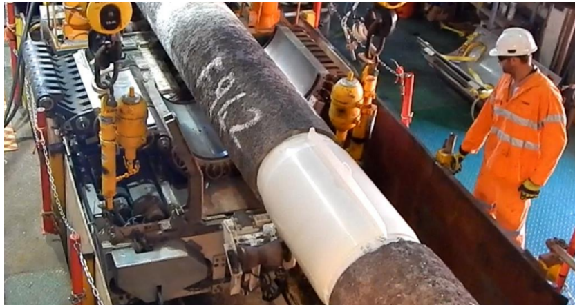
Figure 1.6: Example of concrete weight coating with a field joint of smooth polymeric material
