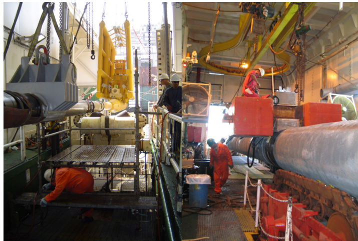
Figure 1.5: Example of inline structures during pipe-laying operations from Smit [20]
