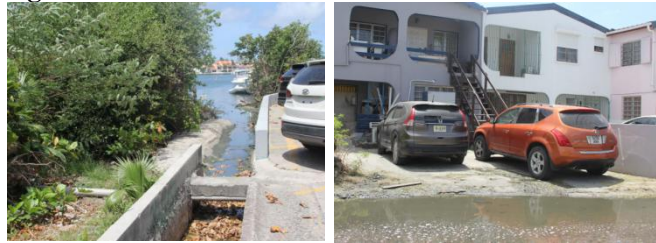
(Left: Open drainage which directly connect the lagoon; Right: Water on the road surface caused by impermeable pavement and bad urban drainage system, photo by author)
