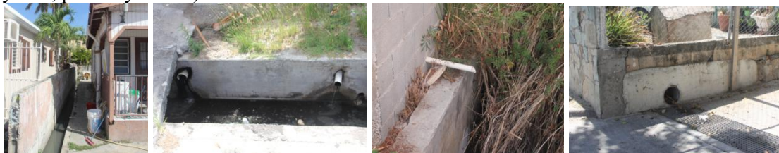
(Residents dig a drain near the house and discharging domestic wastewater or directly to the urban drain, photo by author)
