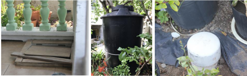
(Cistern, water tank and septic tank hole, photo by author)
