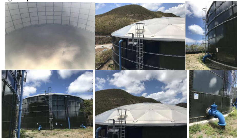
(Picture of water tank, photo by author)
