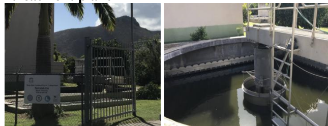
(Wastewater treatment plant A.T.Illidge Road, photo by author)
