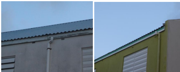
(Meaningless rainwater collection pipe in Belvedere community, photo by author)
