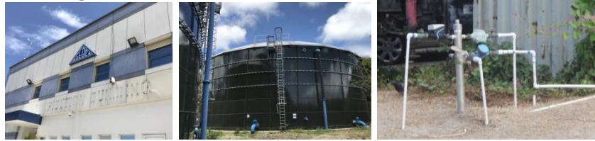
(GEBE office, their water storage tanks and supply pipe, photo by author)
