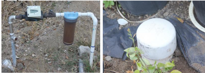
(Left: Filter in this family; Right: the hole of their septic tank. Photo by author)
