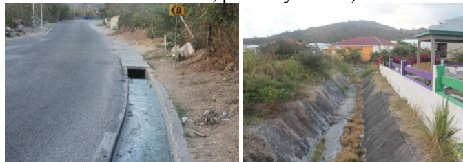
(Drainage near urban roads and in a community, photo by author)
