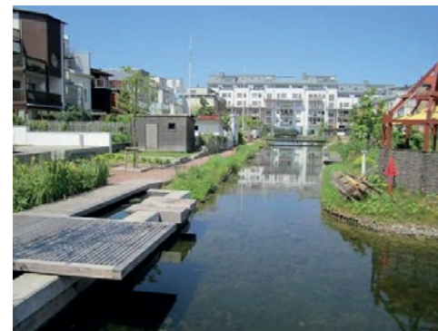
View of permanently inundated SUDS water feature with accompanying community facilities. Image credit: University of Nottingham ( https://blogs.nottingham.ac.uk/blue-greencities/2017/09/01/malmo/ )
