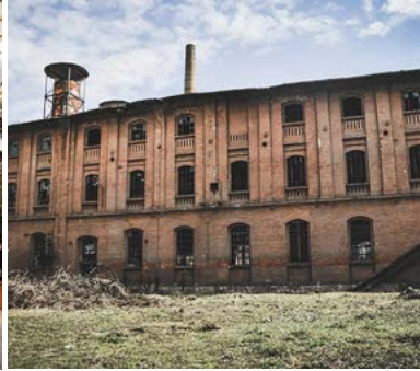
Typical Industrial Building
