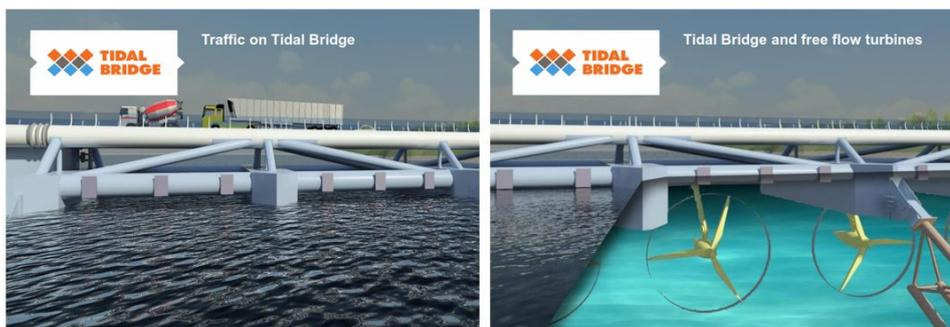
Figure 1.1: The two main functions of the Tidal Bridge: a connection and a power plant (Tidal Bridge, 2018)
