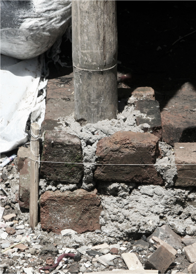
fig. 15. Bamboo column being concealed (van Splunter, M. 2016)
