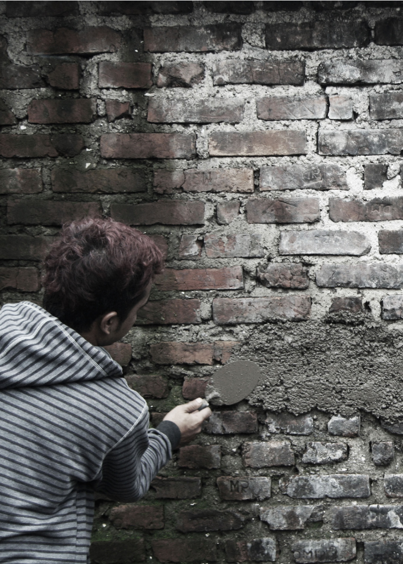
fig. 16. Concrete covering of brick wall (own image, 2016)
