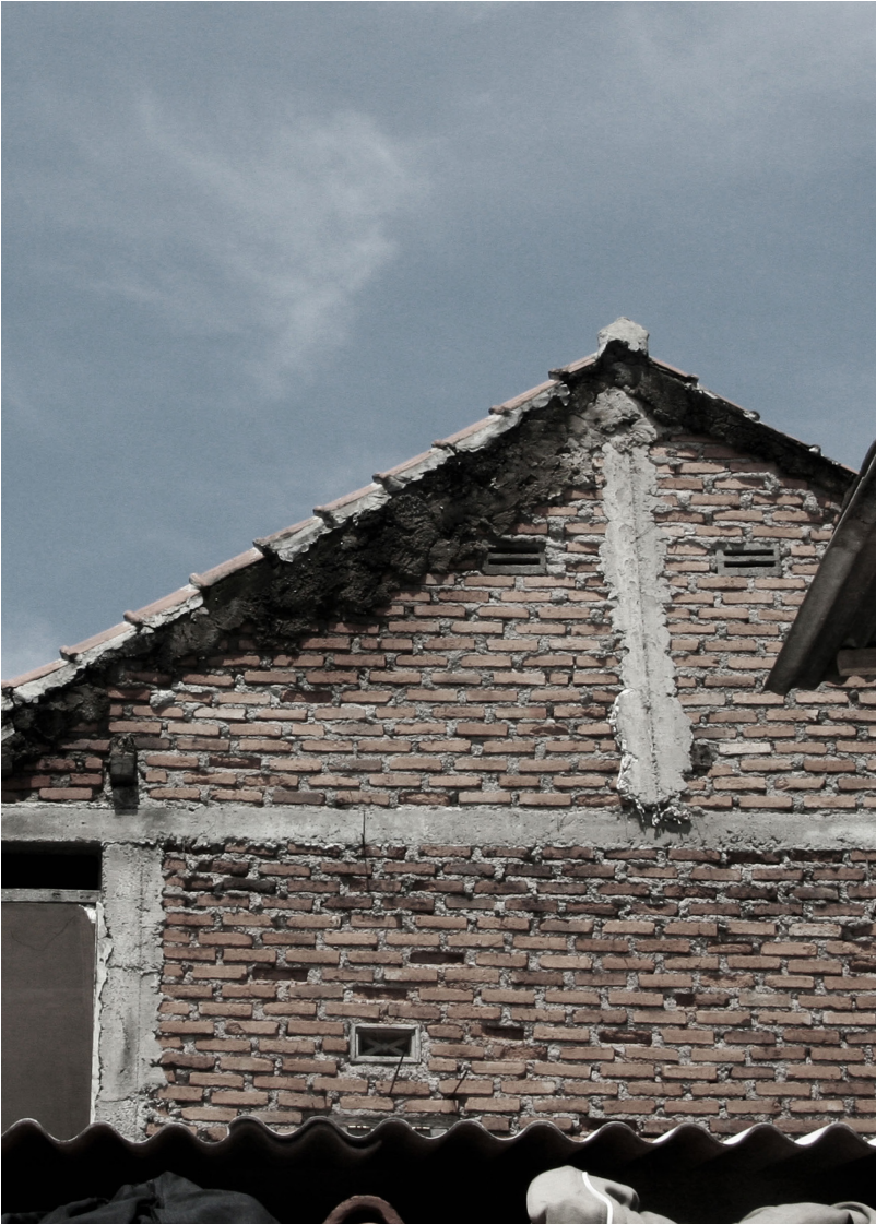
fig. 14: Concrete frame structure (van Splunter, M. 2016)
