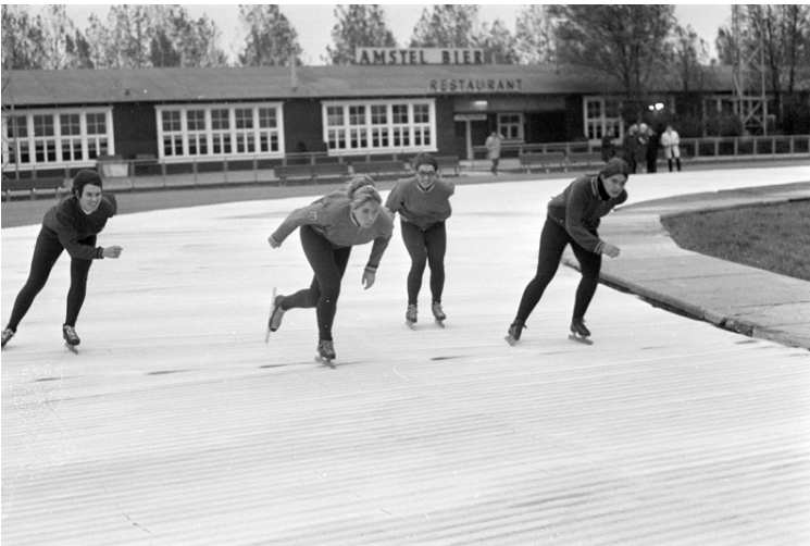
Im. 6.8: The first skating practice at Jaap Eden Baan Amsterdam, October 19th 1967, in the ice are visible pipes, (ANP Foundation)
