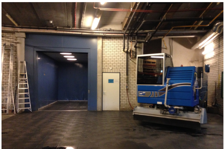
Ice resurfacer parking and snow disposal well in Triavium, Nijmegen, own picture.
