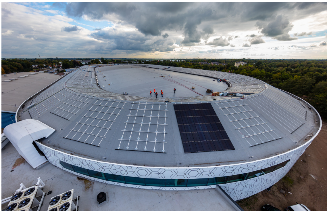
5000 solar panels applied on the roof of Thialf with a capacity of 1,3MW, during the renovation of 2016 (Nuon, 2016).
