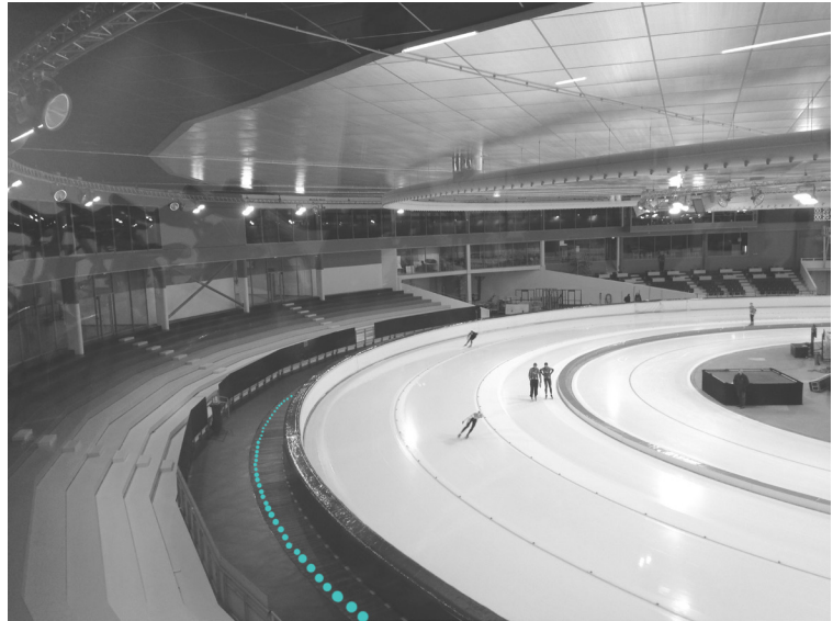
The aircurtain outlets of Thialf, marked in blue, own picture.
