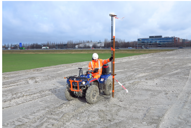
Figure 7.4: A zakbaken placed in to monitor the settlement of a sand body (Roolvink, 2015)
