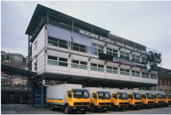
Figure 2.3: Modular-T building in Neuchâtel ( Modular-T n.d.).
