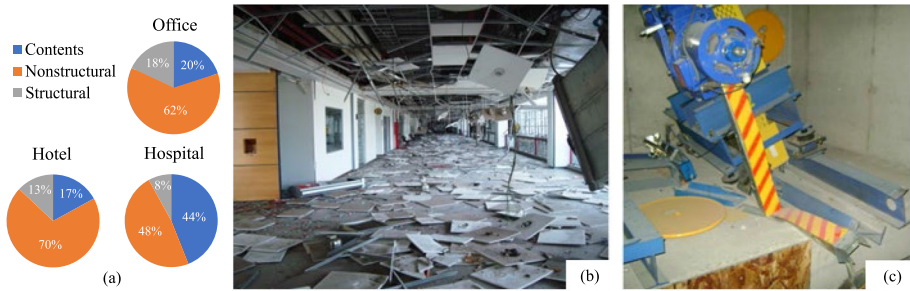
Fig. 1 a Typical distribution of structural and non-structural parts of buildings (modified after Taghavi and Miranda 2003). Damage to NSCs in Santiago International Airport, Chile, after the 2010 Maule earthquake: b damaged ceilings; c damaged lift motor (pictures from Cowan et al. 2011)
