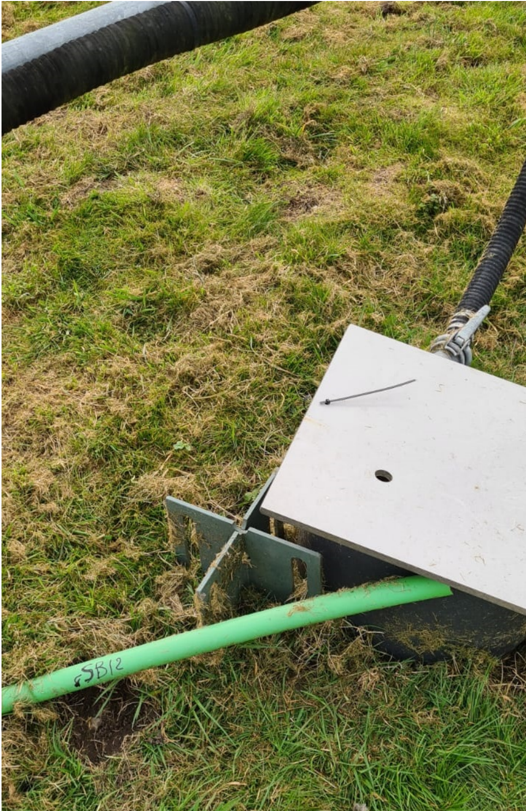
Figure A.9: Example of ground settlement beacon obscured by soil, vegetation and other objects. Beacon is in the bottom left of the photograph, as marked on the green tube.
