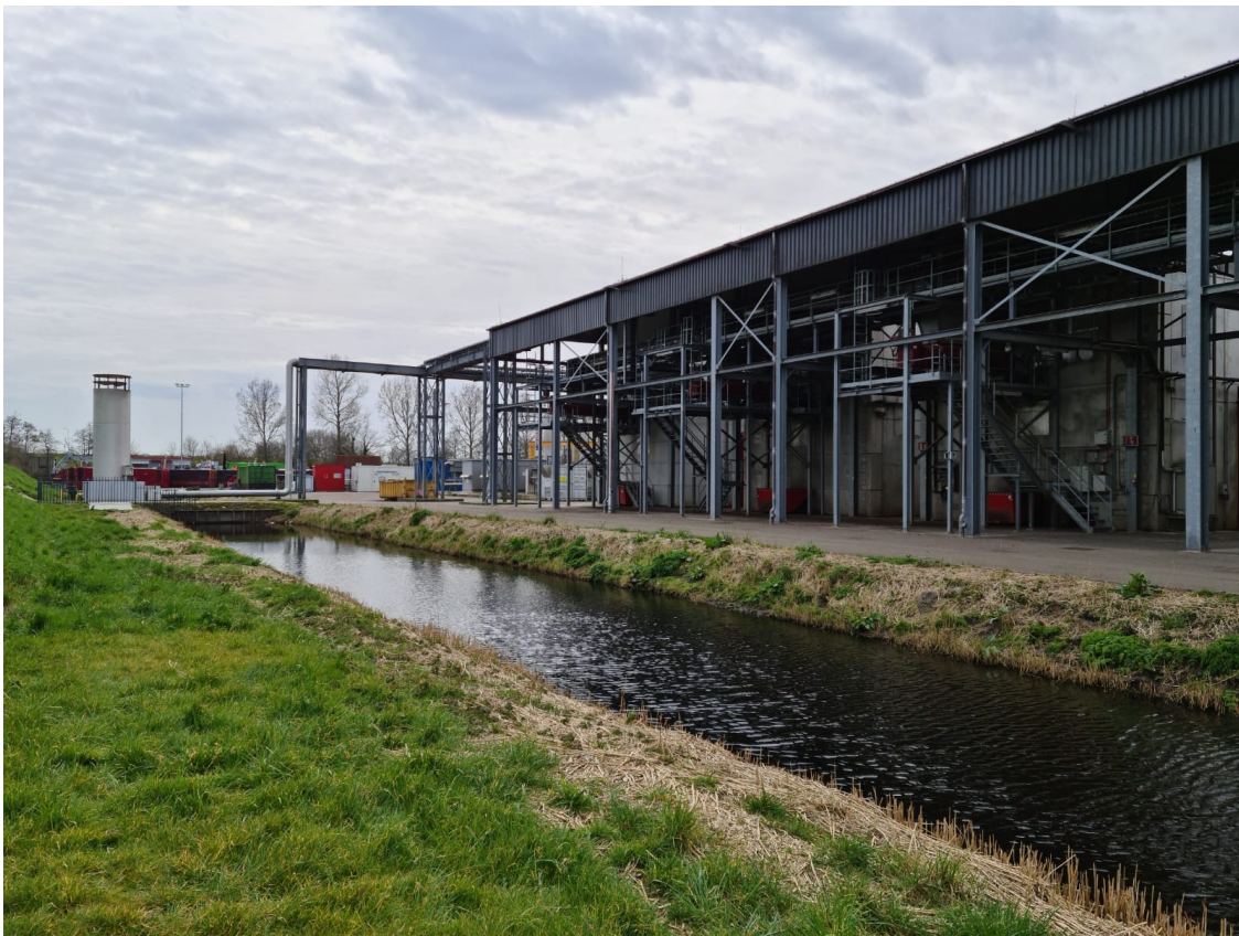
Figure A.6: Structural elements of the building on the right side of the photograph used for the registration process.
