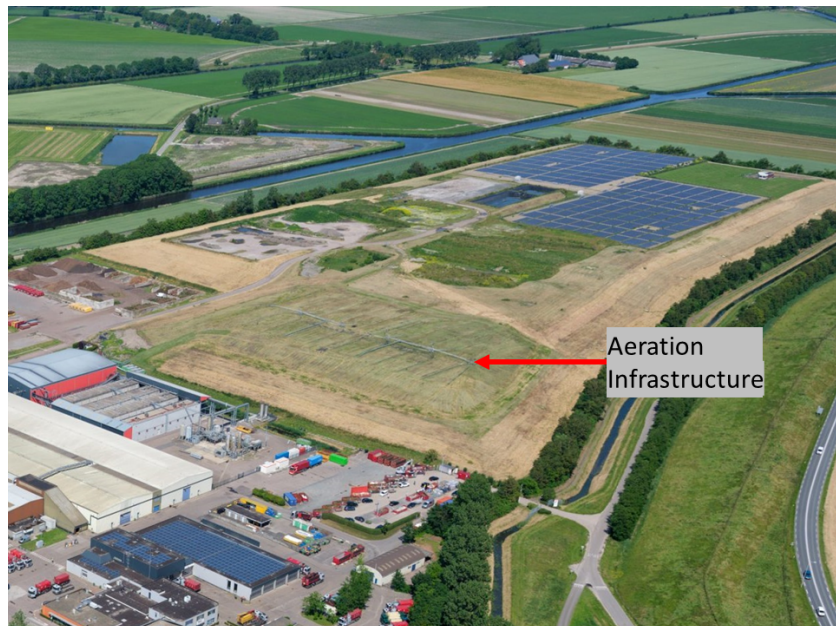
Figure 2.2: Side on perspective of the Wieringermeer landfill, image taken from the SW direction by Afvalzorg.
