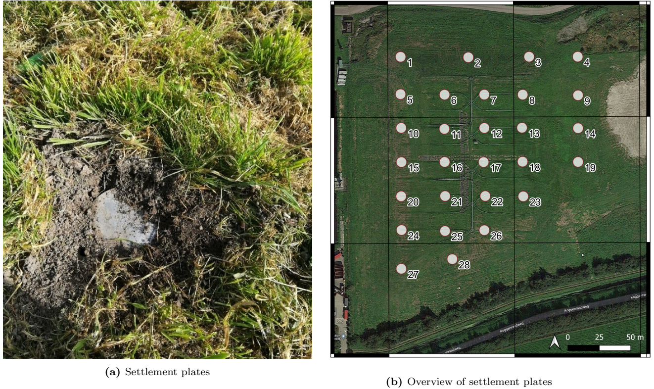
Figure 3.3: Photograph of a settlement plate installed on the landfill and an aerial overview of all 28 plates.
