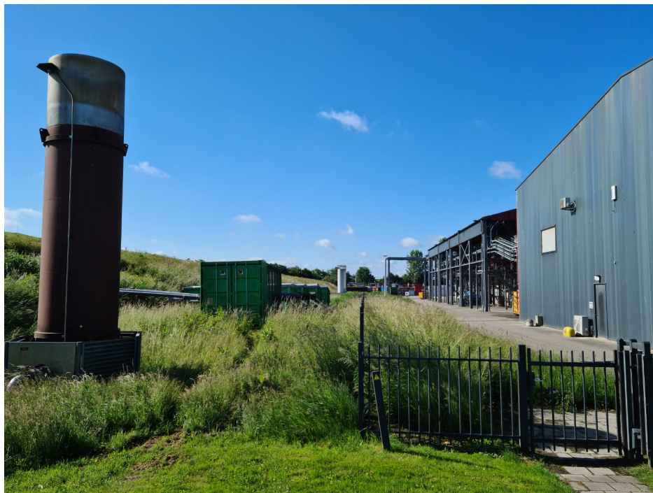
Figure A.7: Smokestack on the left, and containers in center of the photograph used for the registration process.
