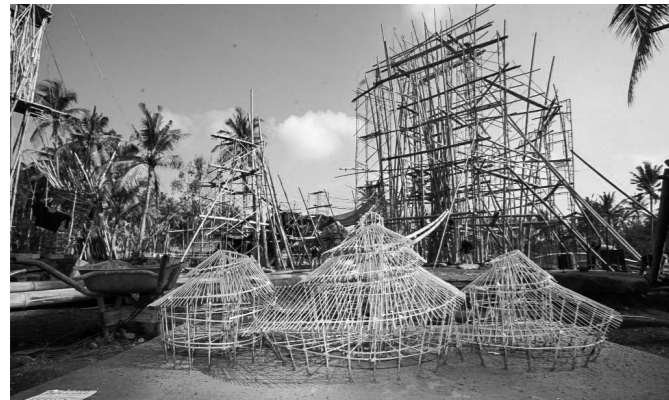
Figure 39-Bamboo scale model as reference for construction.
