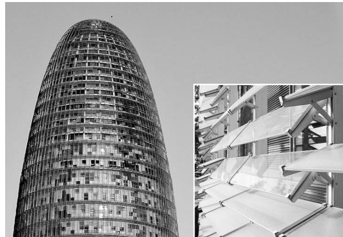
Figure 77-Agbar Tower façade elements.
