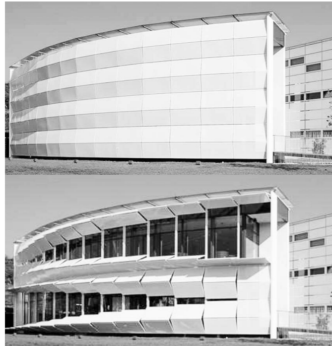
Figure 69-Kiefer facade shading elements.
