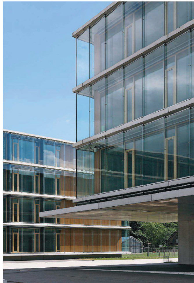
Figure 158-Exterior view from case study building.
