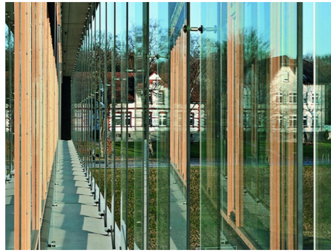
Figure 159-View from the façade cavity of the case study building.
