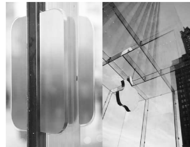
Figure 15-Apple store connection detail.
