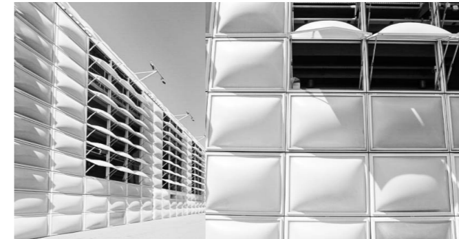
Figure 73-St Jakob Park Stadium façade detail.
