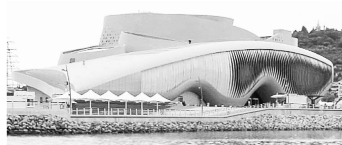
Figure 43-One Ocean Pavillion with open and closed louvers.
