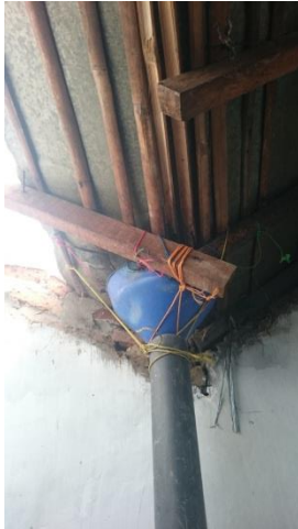
Figure 61: Guttering used in the rainwater harvesting system. The gutter is connected with a funnel to the roof, and afterwards the water is transported with a pipe towards the tank.
