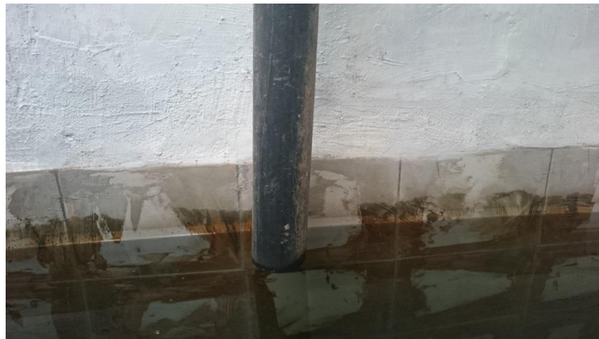
Figure 61: Guttering used in the rainwater harvesting system. The gutter is connected with a funnel to the roof, and afterwards the water is transported with a pipe towards the tank.
