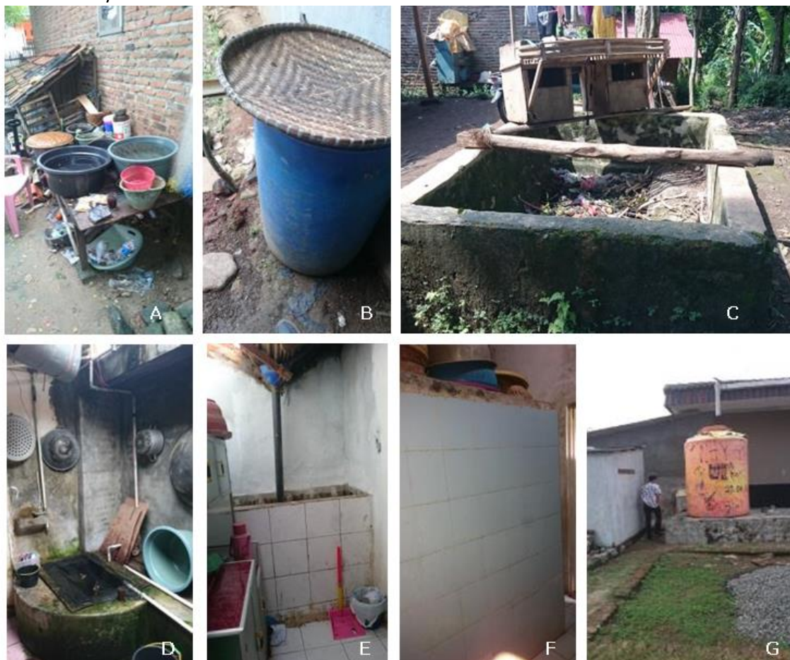
Figure 27: Individual rainwater harvesting systems that are found in kabupaten Serang.
