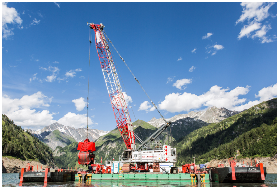
Figure 5.4: Example of a grab dredge, used to dredge the Luzzzone reservoir (Liebherr, 2017)
