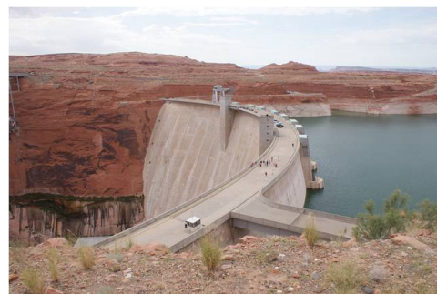
Figure 1.1: Example of a reservoir.
