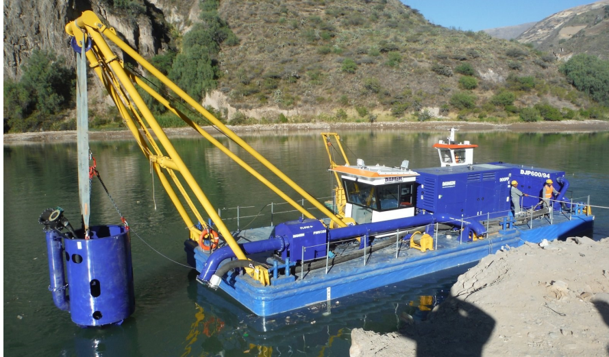
Figure 5.7: Example of a pump dredge, used to dredge a reservoir in Peru (Damen, 2016)
