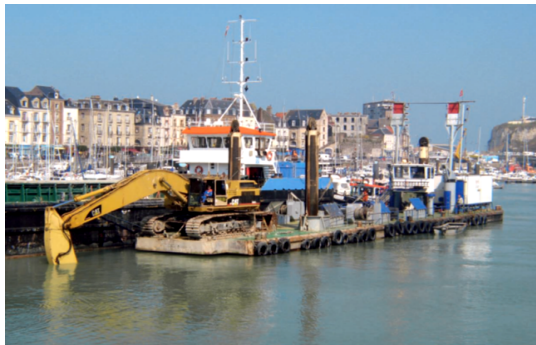
Figure 5.5: An excavator mounted on a pontoon with spuds (Baggerbedrijf de Boer B.V., 2014).
