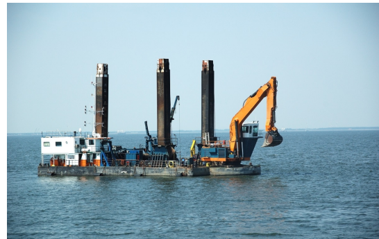
Figure 5.6: An example of a backhoe dredge, mounted on a barge (Van Loon Maritime Services B.V., 2017).
