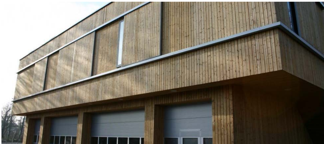
Figure 119: Insulating shutters at the Gemeentewerf in Amstelveen by Isoluijk B.V. (Isoluijk)
