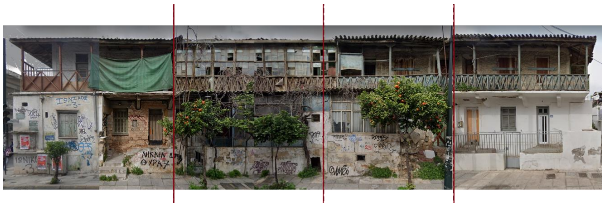
Figure 17: Combined views from the street of 16 apartment houses, poorly maintained in 2014. In this case, the building is probably neglected for years apart from the flat on the bottom right, which shows more care. Here the original railings have only been replaced on the left unit. In the corner
