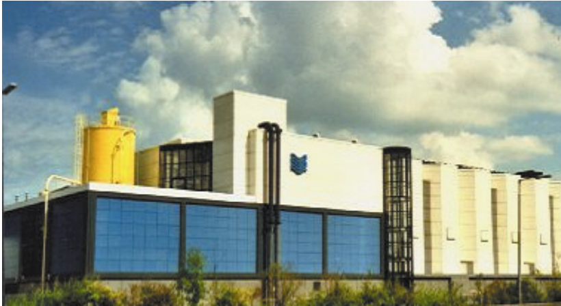
Figure 5.5 WTP Reijerwaard, Hydron ZH
