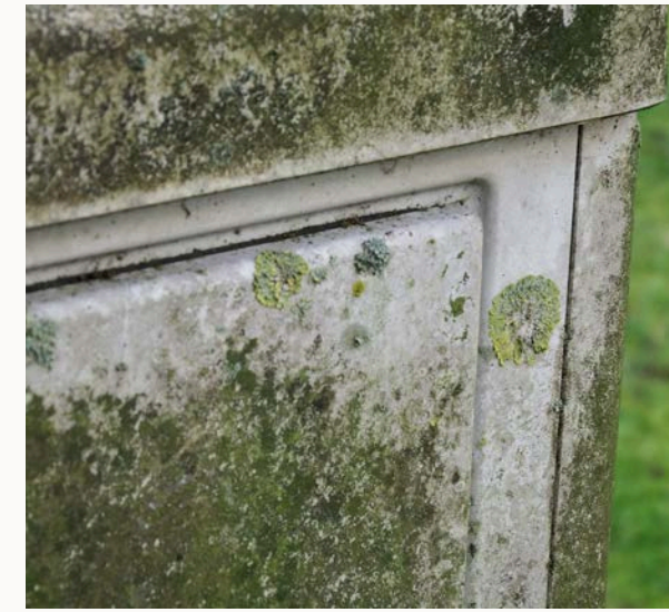
OBS. 01 — BIOFILM ON SMOOTH SURFACE
