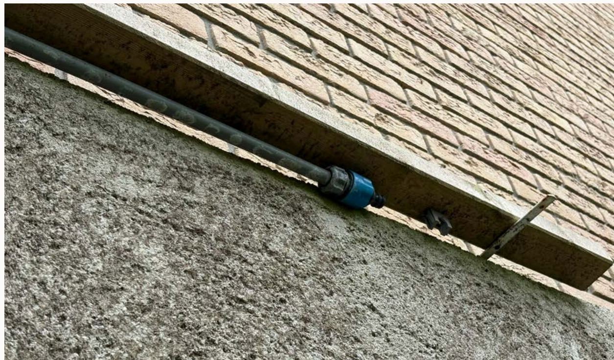
Fig. 1.12 — Respyre Porous Concrete Coating Utilizing Temporary Irrigation Infrastructure
