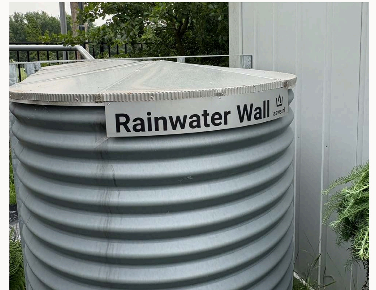
Fig. 5.28 — Rainwater buffer in use at The Green Village.
