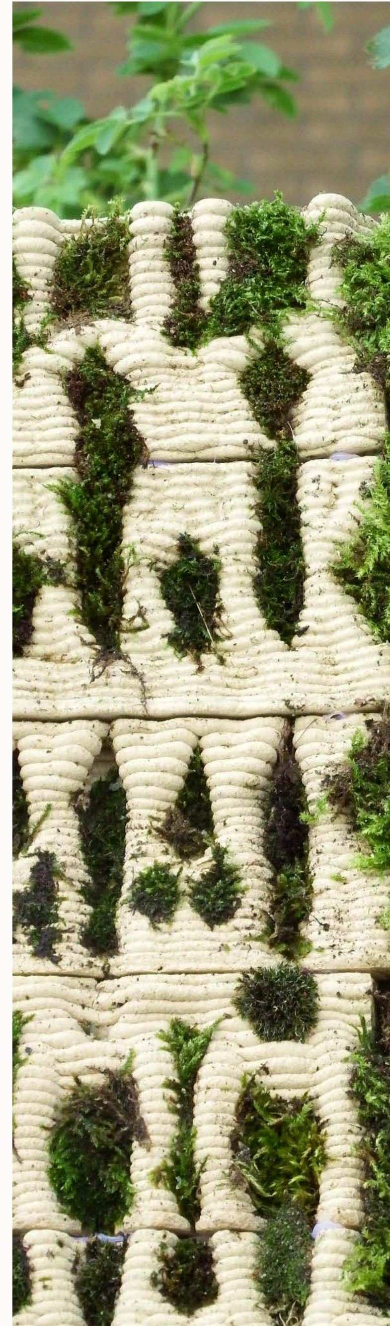
Fig. 6.4 — Close-up: moss pressed into the porous valleys where water is held, while the raised peaks stay clear.
