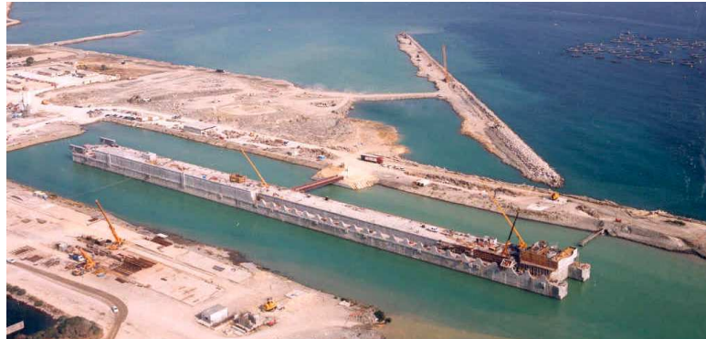
Figure 8.2 The dry-dock in which the Monaco floating breakwater was built
