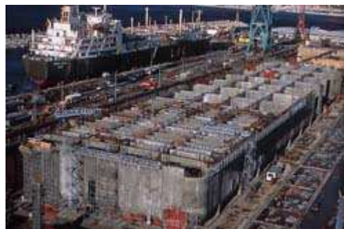
Figure 8.1 The N’Kossa barge under construction in a dry-dock
