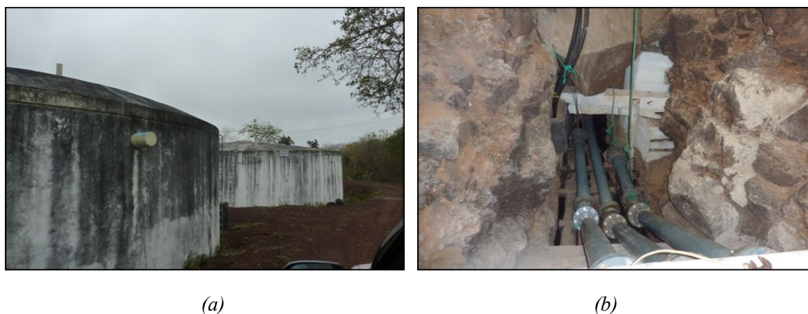
Figure 3.3-Pictures of (a) Storage tanks and (b) three pumps installed for extraction of brackish water at "La Camiseta".
