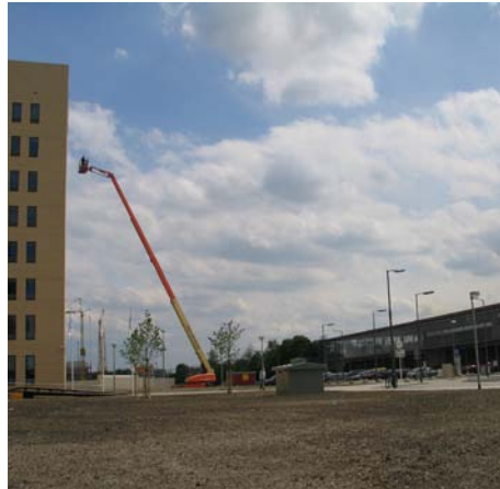
Figure 2.3.17 Vacant Space Outside of North Gate of Station
