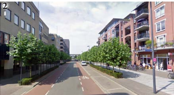
Figure 4.2.12 Link 2 - the main link from station connecting other parts of the transformed area.
