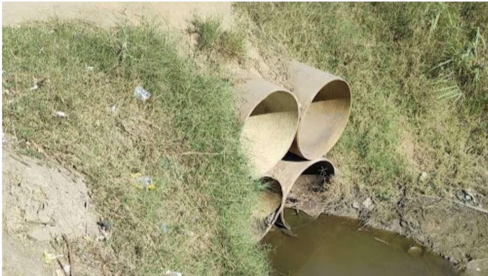
Figure 2.1: Bridge made from local materials in Chota, Beira (picture by author)
