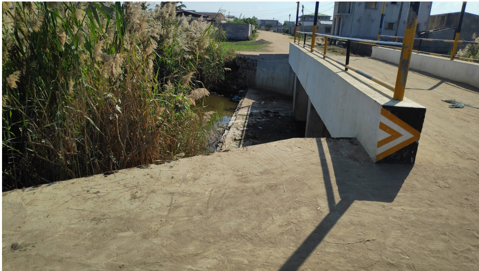
Figure 2.8: Bridge in the drainage system in Chota, Beira (picture by author)
