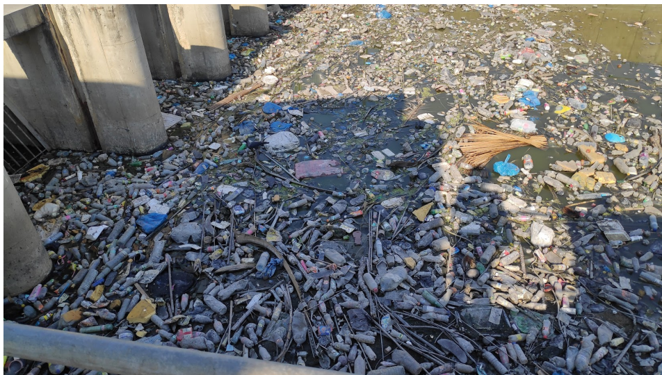
Figure 2.6: Waste accumulating at a bar screen in Beira (picture by author)
