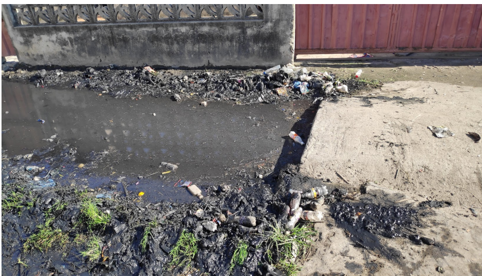
(a) A concrete bridge in a canal in Munhava-Matope, Beira (picture by author)
