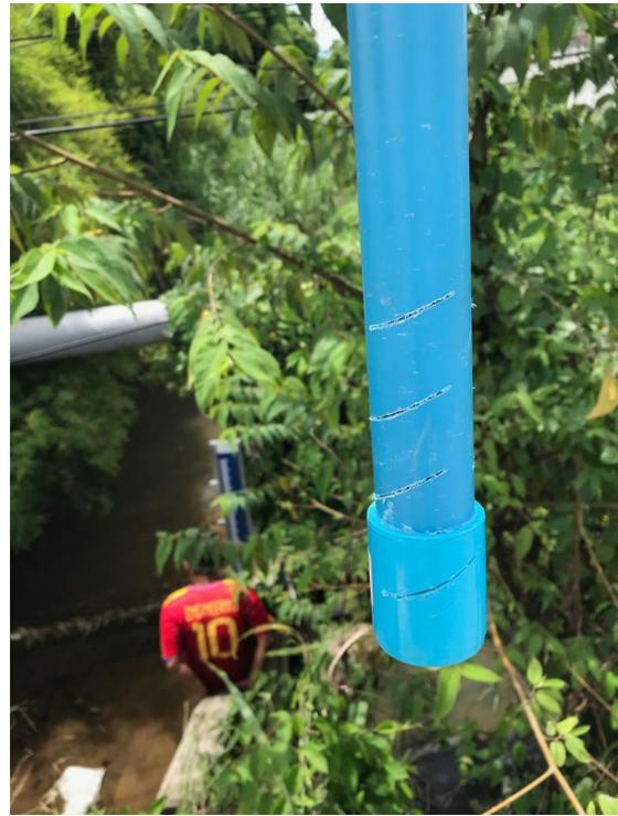
Picture 9: Monitoring tube for Diver.
