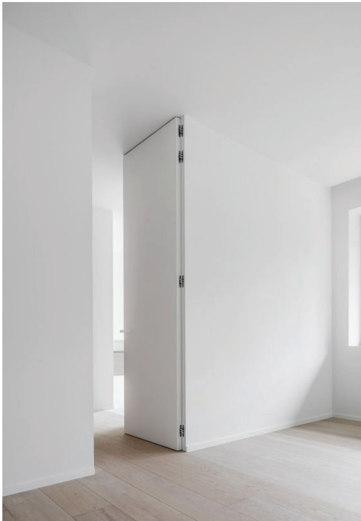
TECTUS Hidden Hinge for panel wall
