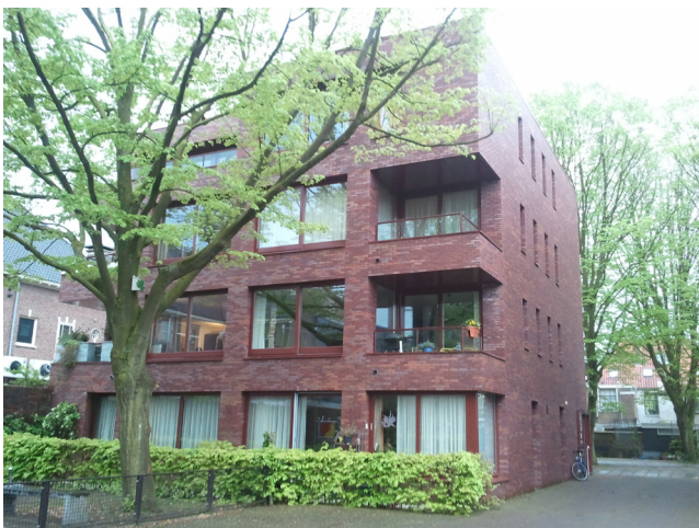
Fig. 104 Reference modern, Dutch architecture (Schuttersveld, Delft) Geurst & Schulze architecten (author, 2012)
