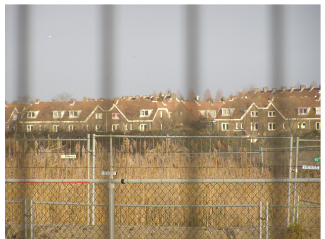
Fig. 44 Van der Pekbuurt behind construction fences (author, 2011)
