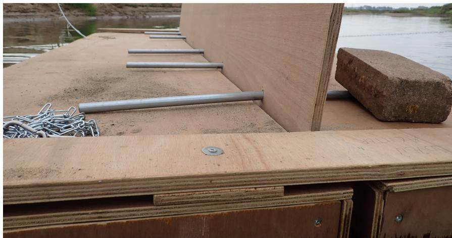
Figure 3.5: Screen mounted on the floating body using metal pipes
