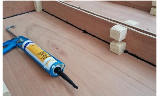
Figure D.12: Prohibition of leaking by applying sealant
