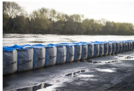
Figure 3.19: Sand bags are an example of temporary barriers (source: HESCO, 2016)
