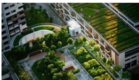
Figure 3.30: Green roofs and green spaces are examples of delaying the rainwater runoff in urban areas (source: Hendriks, 2017)
