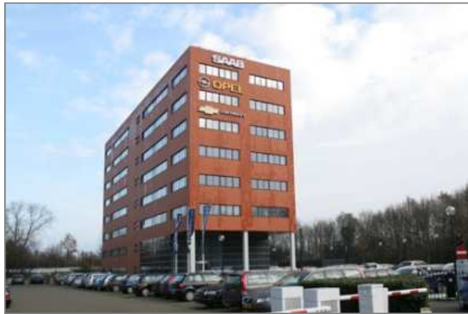
Figure 5.11 Building Opel, Westerhage
