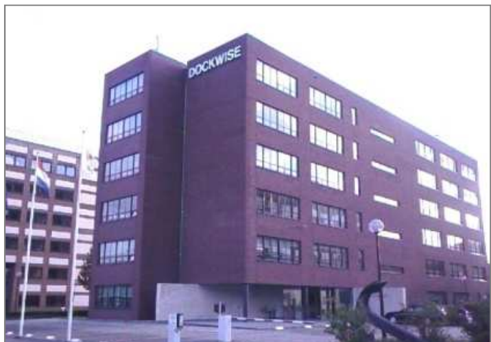
Figure 5.2 Building Dockwise, Westerhage
