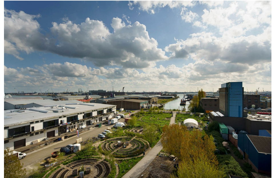
Industrial area around Keilepand, Keilekwartier
