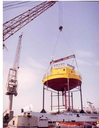
**Figure 2.4** Vertical axis tidal stream turbine: Kobold [©LoStrettoNecessario.net] [7] .
