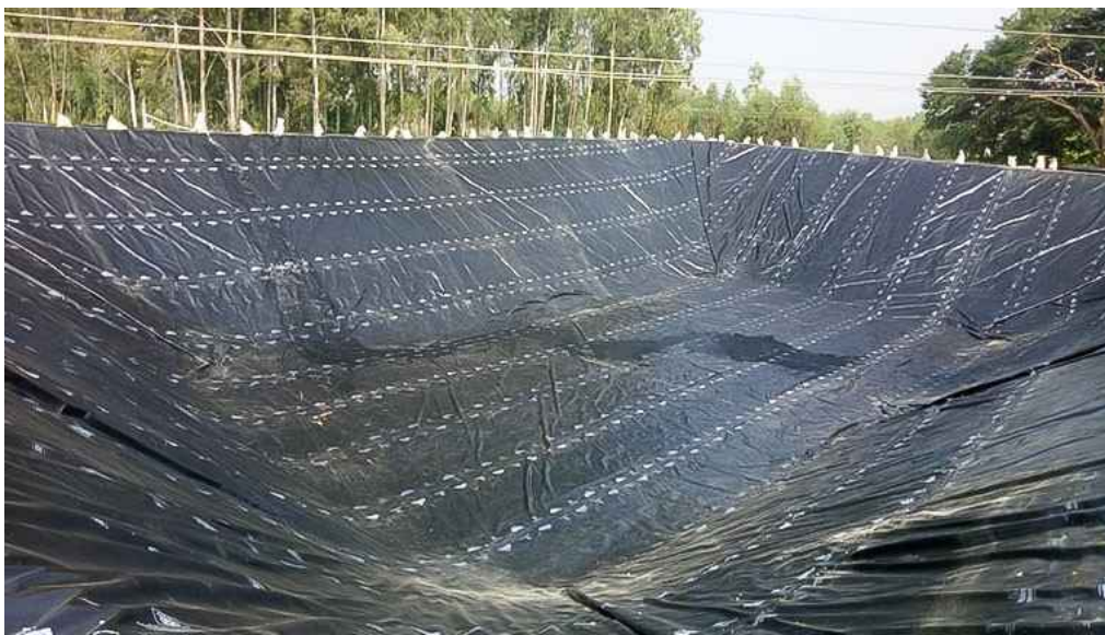
Figure 3.2: Illustration of a geo-membrane representative, proposed for mine pond rehabilitation [63]
