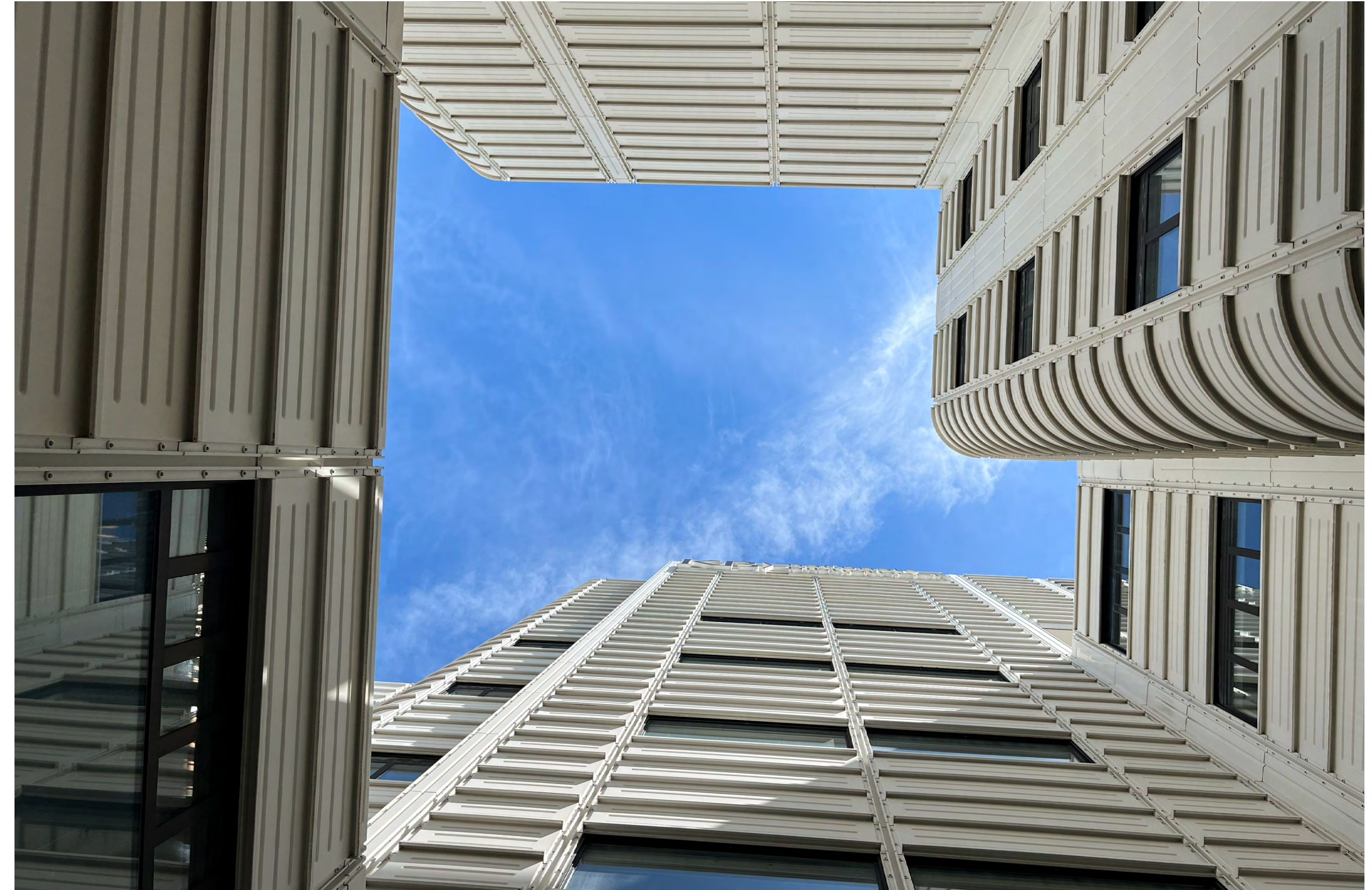
'rain coat' facade (Own image)
