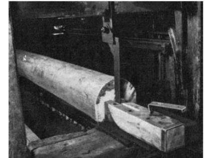
An example of an early frame saw cutting log into dimensioned timber (source: Finsterbush 1987)
