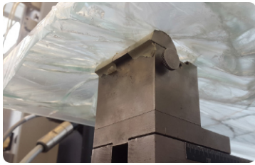
Image 6: panel penetrated by the support
