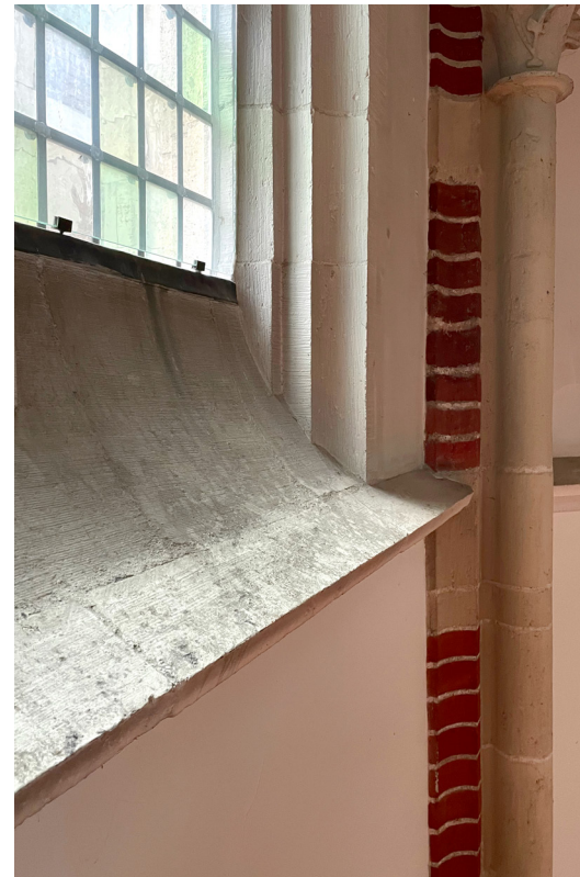
THERMAL BRIDGE REDUCED WALL THICKNESS
