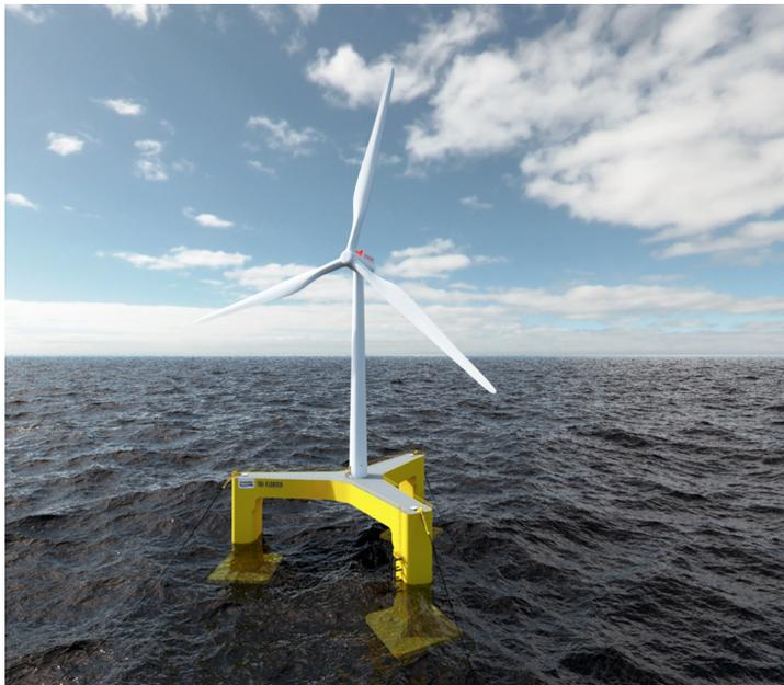
**Figure 4.1:** Artist impression of the GustoMSC Tri-Floater with the 5MW NREL reference wind turbine positioned in the center, in irregular waves.
