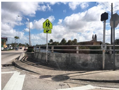
Image 64. Lack of pedestrian connections. Source: author
