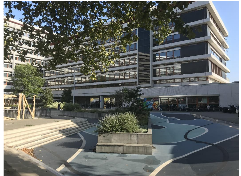
Image 15. Urban landscape as infrastructure: Water Square in Rotterdam by the Urbanisten. Source: author.
