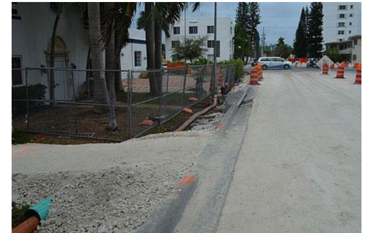
Image 4. Elevated road and sidewalk public works in a residential area of Miami Beach. Source: https://www.yaleclimateconnections.org/2017/05/miami-beach-is-spending-millions-to-hold-back-the-sea/
