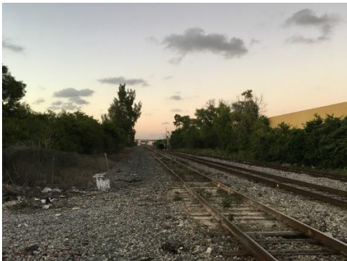
Image 61. Decayed buffer zones. Source: author
