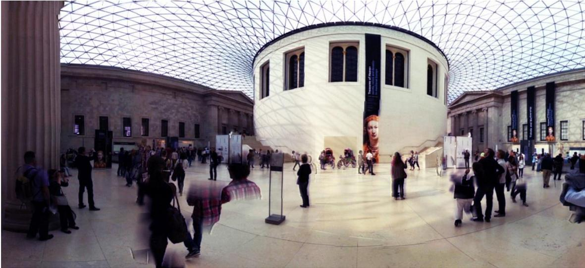
**Fig. 51: A triangular grid-shell made of steel provides the roof structure for the courtyard of the British Museum in London**
