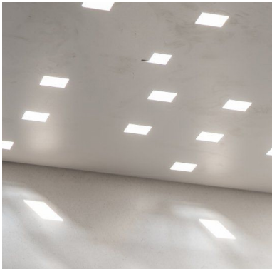
ceiling plastered with skylights
