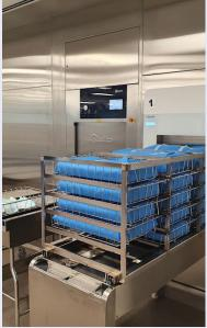
Here the nets come out in the sterile part. The CSD employees will check whether devices have come out fully dry and check whether the autoclave program has run appropriately.
