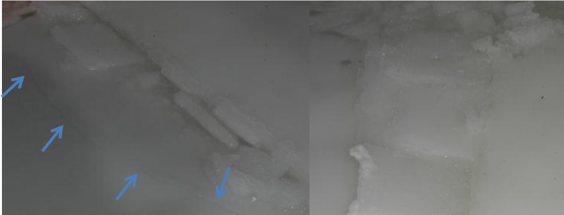
Figure 2-19: Left: a large crack prior to arrival of model, its length is roughly 100 meters. Right: the rubble in the gap that behaves rather weak.
