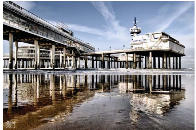
Rebuilding of the Pier (Scheveningen) by ABBT.
