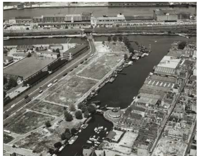
Kattenburg is completely empty and ready for a new urban plan. This picture is made in 29 juni 1972.
