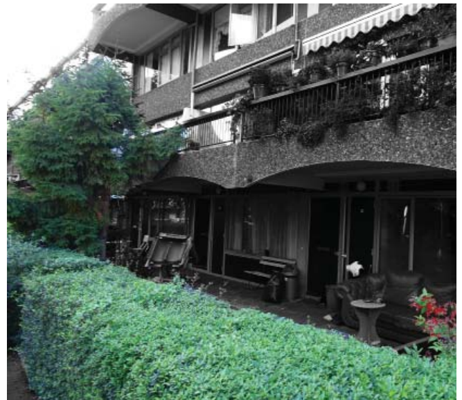
Facade of ground level housings which have small front garden
