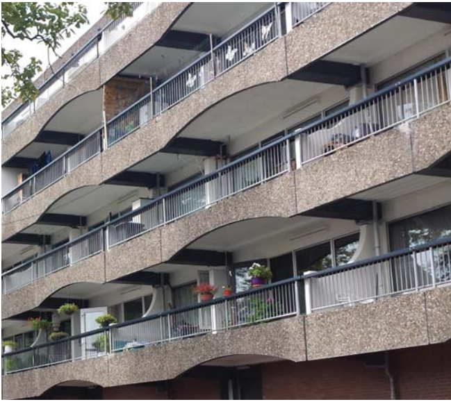
The balconies have a rough concrete surface
