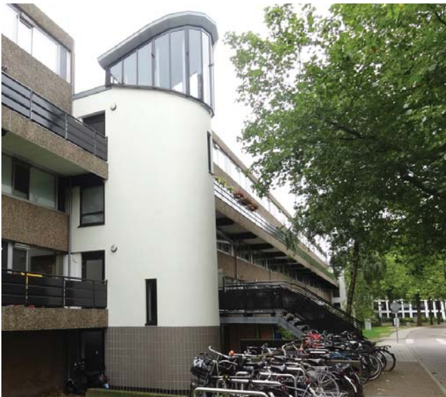
The staircases are in plastered towers
