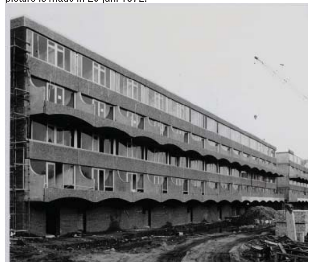
The first new buildings of Kattenburg designed by ABBT architects.
