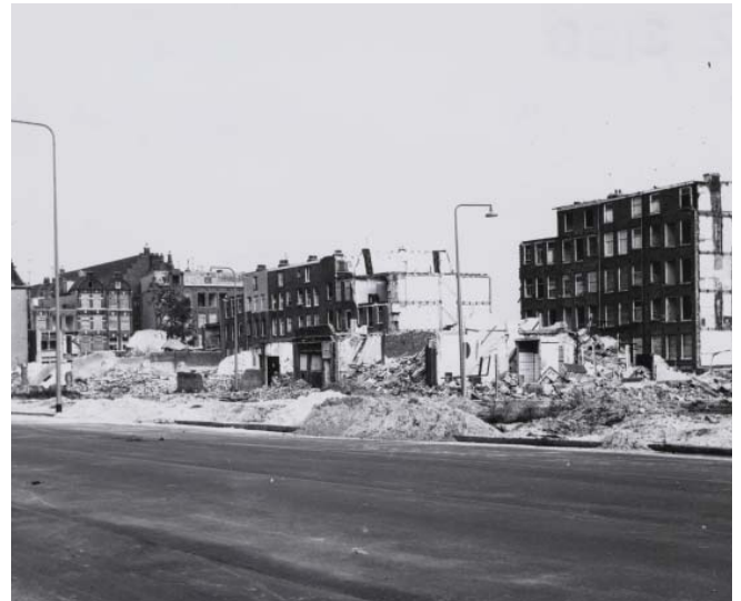
Demolishing of Kattenburg
