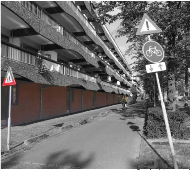
Facade of storage part
