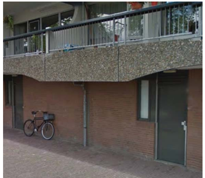
The basements have a brick façade
