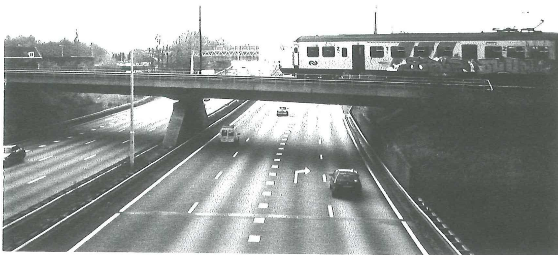
Krappe overspanning viaduct NS Noorder- bocht
