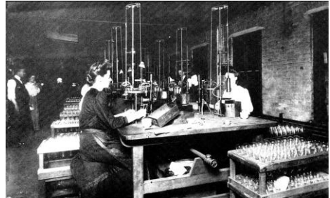
Figure 146: Westinghouse employees manufacturing stopper lamps for the Columbian Exposition (1893)
