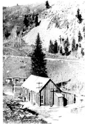
Figure 137: Powerhouse of the Ames Hydroelectric Generating Plant
