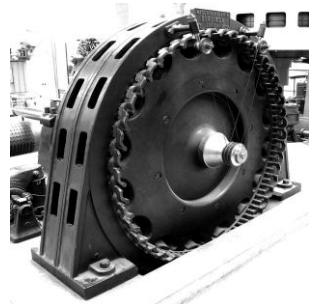
Figure 133: The Oerlikon 220 kw generator used in Lauffen (1891)
