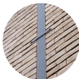
Aluminium rainwater pipe
