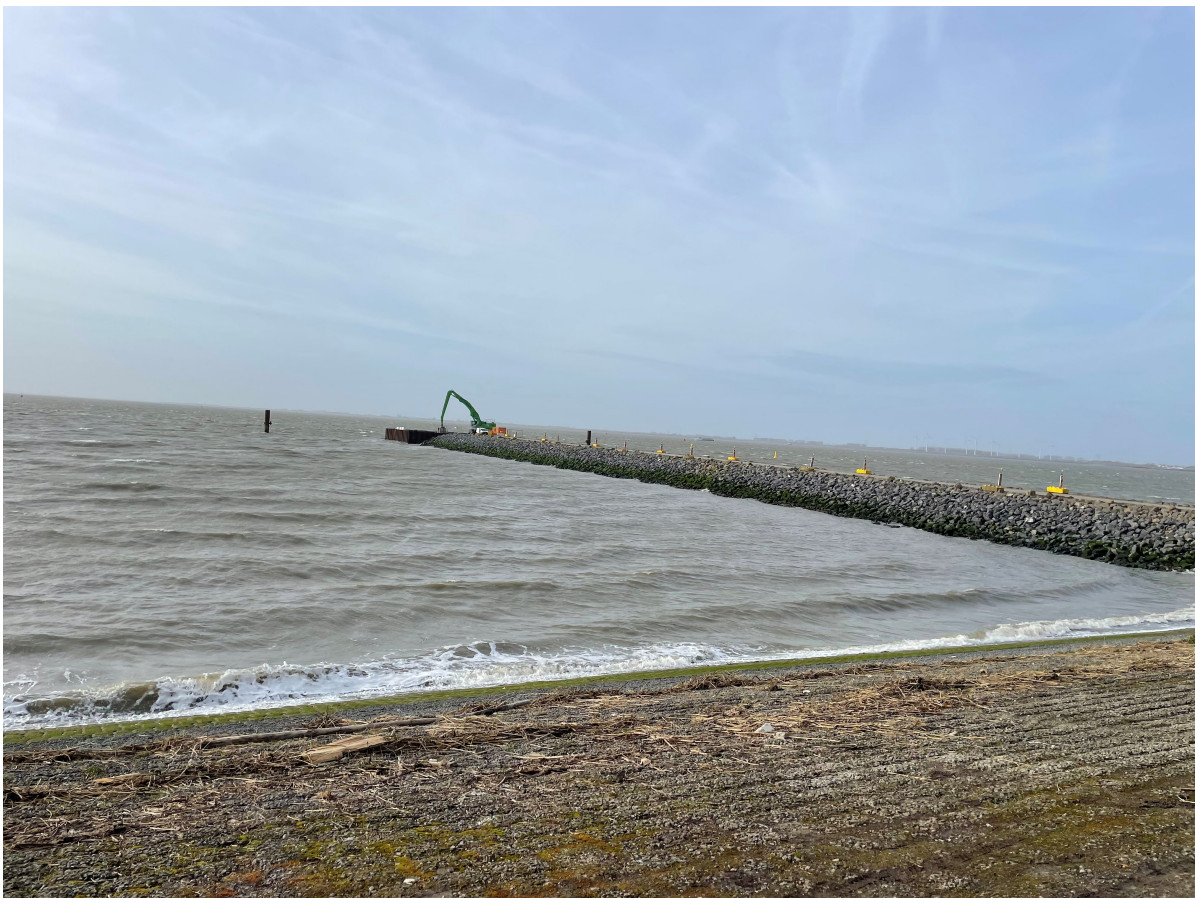
Figure G.1: Temporary dike and quay wall at Hansweert
