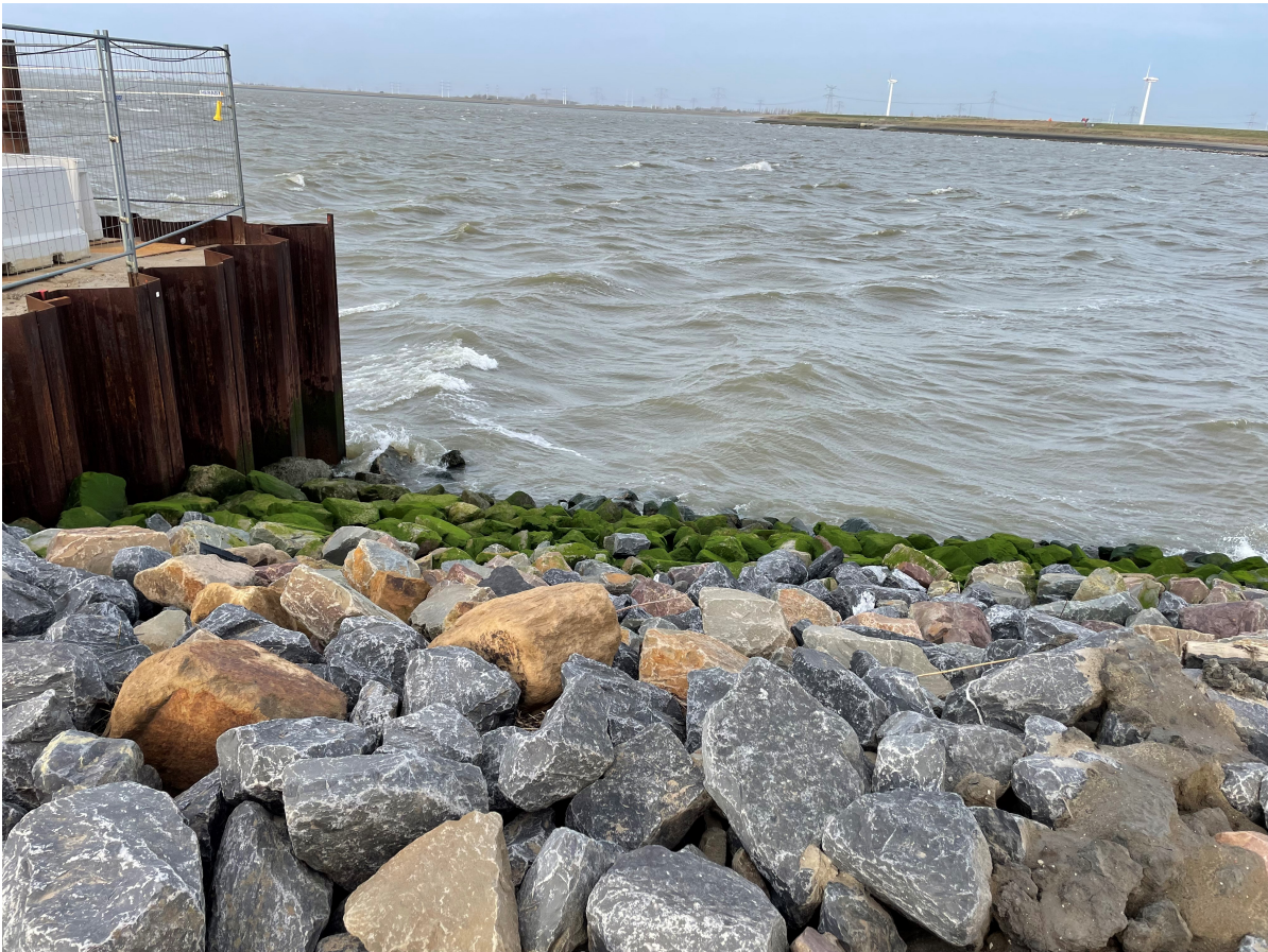
Figure G.2: Transition from dike to quay wall at Hansweert
