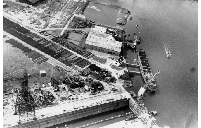
5.3 Docks and finishing quays Steel plates were stored along the streets.
