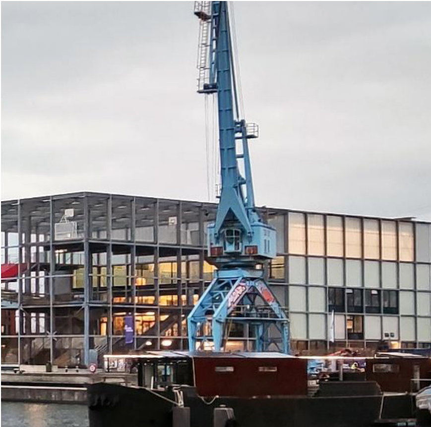
6.14 Shipbuilding Crane In 'Oude Dokken' in Gent
