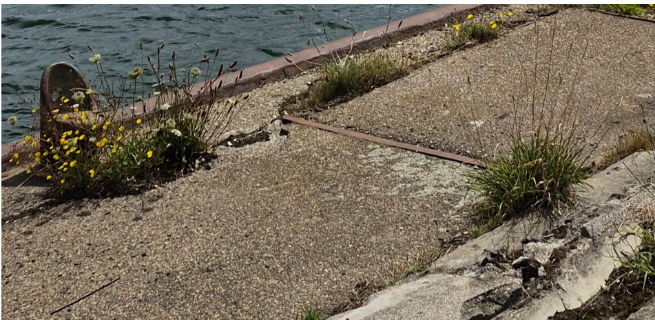
6.7 Existing materials in the 'Scheldekwartier' in Vlissingen
