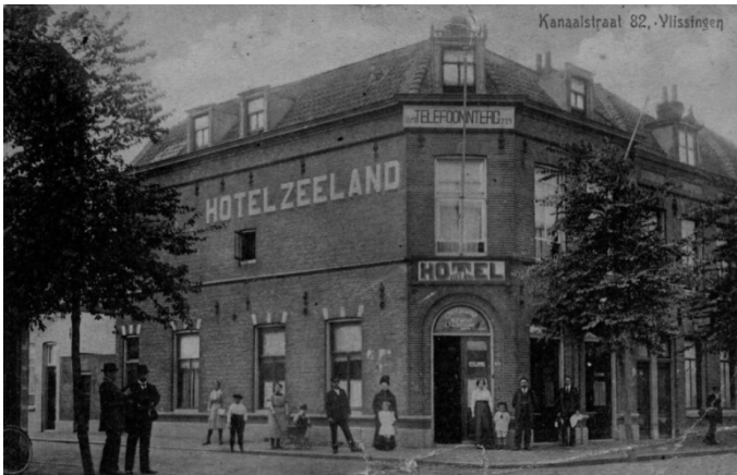
5.6 On of the many hotels, representing the proximity of the station
