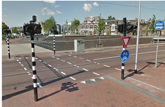
Figure 2.1: Pedestrian/cycling crossing with flashing lights in Delft, the Netherlands Source: Google Earth StreetView
