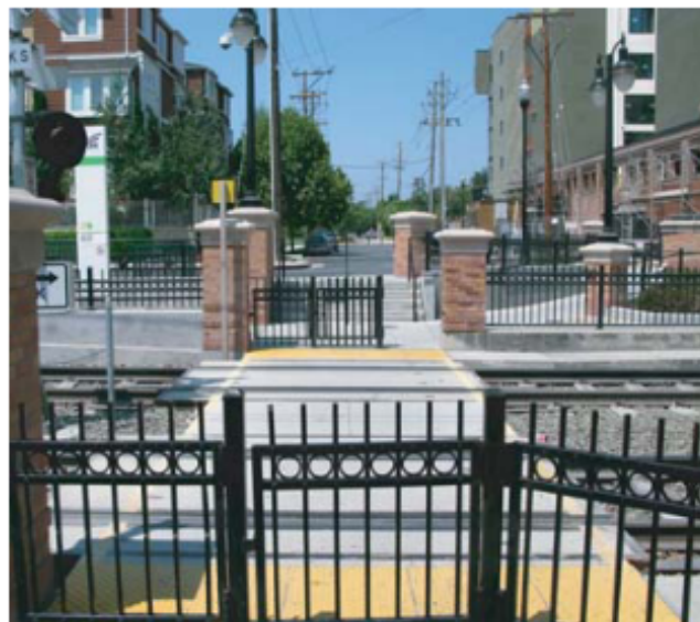
Figure 2.2: Pedestrian crossing with swing gates in San Jose, USA Source: Cleghorn et al. (2009)
