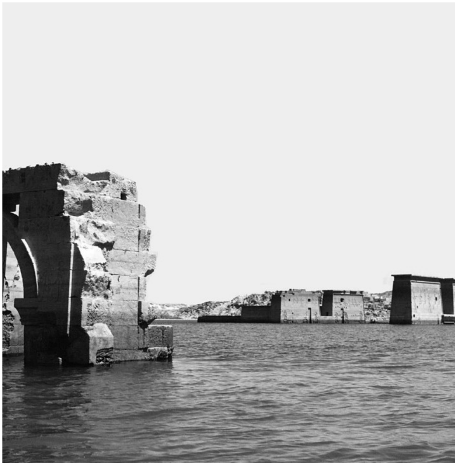
Island of Philiae and Temple of Isis (EG), under water due to the construction of the Aswan Dam (1960-70). In 1968, the temple was dismantled and rebuilt on a neighbouring island.
