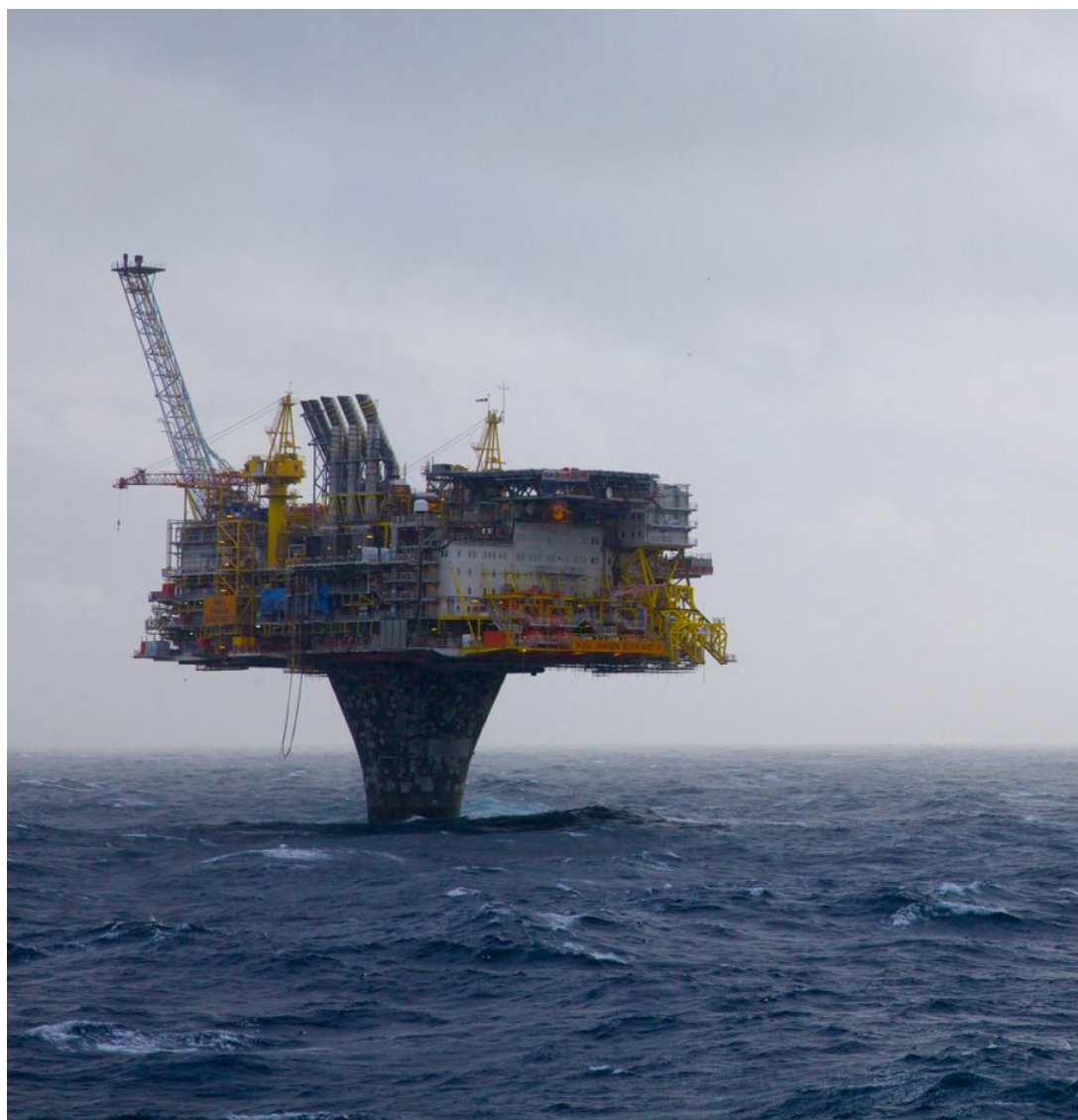
Draugen Oil Field and Platform, Norwegian North Sea (NO), 1993.
