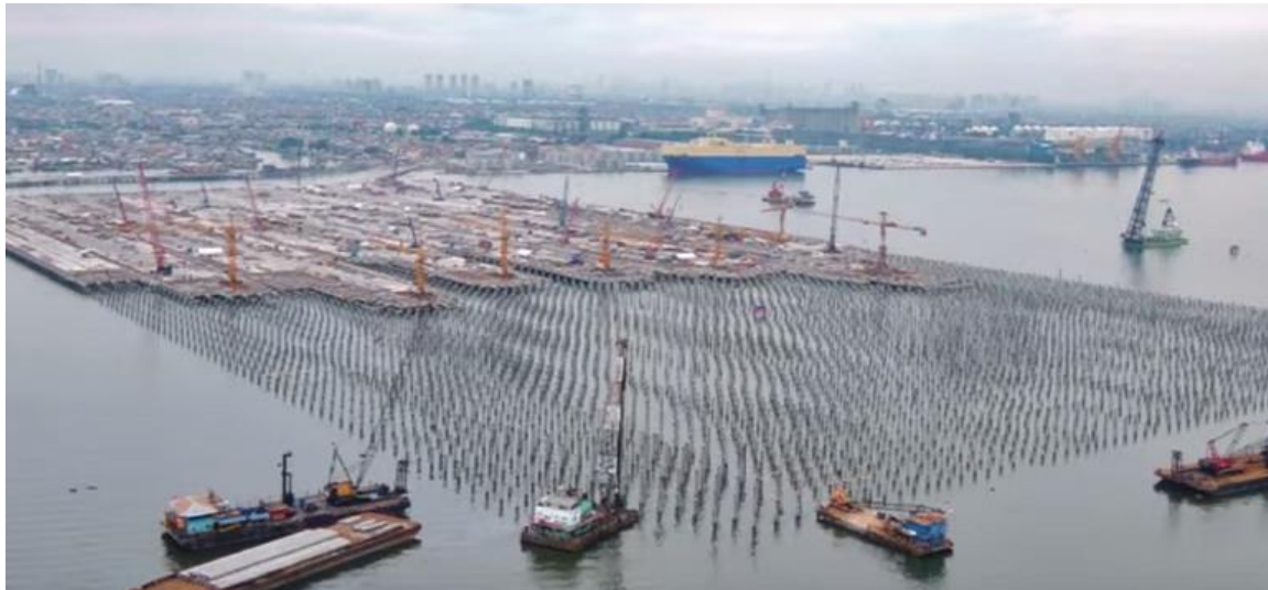
Figure 42 New Priok development Port of Tanjung Priok, Jakarta ( https://www.dutchwatersector.com )
