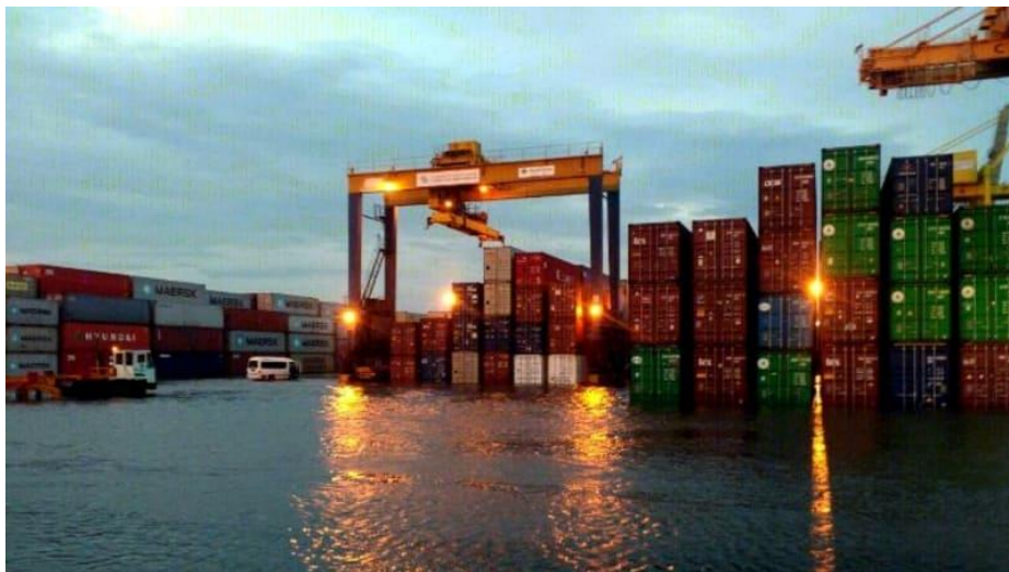
Figure 24 Port of Semarang (Java, Indonesia) flooding of the container terminal ( www.zonamagz.com )
