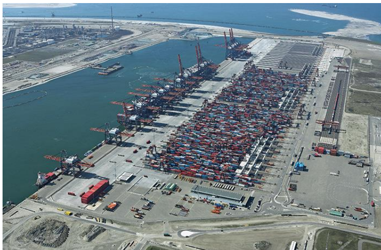
Figure 43 Euromax Container terminal Rotterdam ( https://www.portofrotterdam.com )
