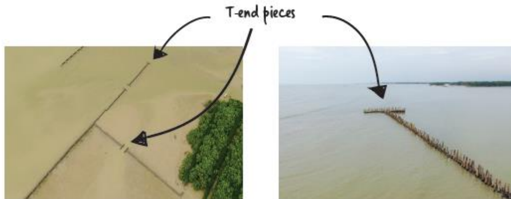
Figure 56 T-shaped ends at openings and at the end of each longshore structure (Ecoshape Demak, 2018)
